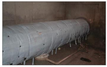
**Application: Steam Service Manhole Expansion Joint & Pipe** Thermal Design: LT550LFP-HS-1 1/2" Thickness
