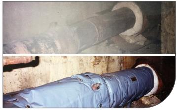
**Application: Steam Service Manhole Expansion Joint & Pipe** Thermal Design: LT550LFP-HS-1 ½" Thickness
