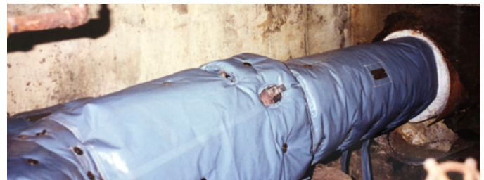
10” Piping / Expansion Joint District Heating - Manhole (Confined Space)
