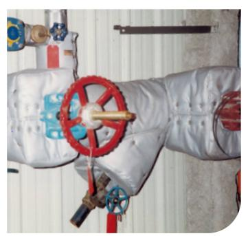
**6" BACK FLOW PREVENTER** Blanket Design: LT450SS Fastener: Stainless Wiretwist
