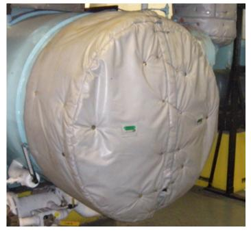
**CHILLED WATER HEAT EXCHANGER HEAD** Blanket Design: LT250VP Fasteners: Velcro Flaps / Stainless Steel Wiretwists
