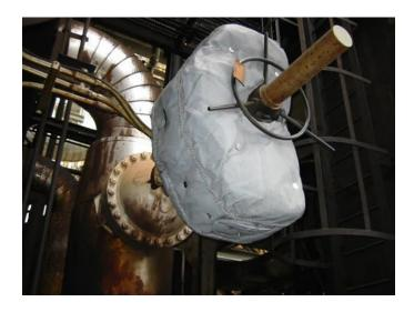
**Leak Accommodations:** To accommodate a leak and detect its origin, blankets will have a low point stainless steel drain grommet or the design will incorporate a mating seam at the lowest point of the blanket.
