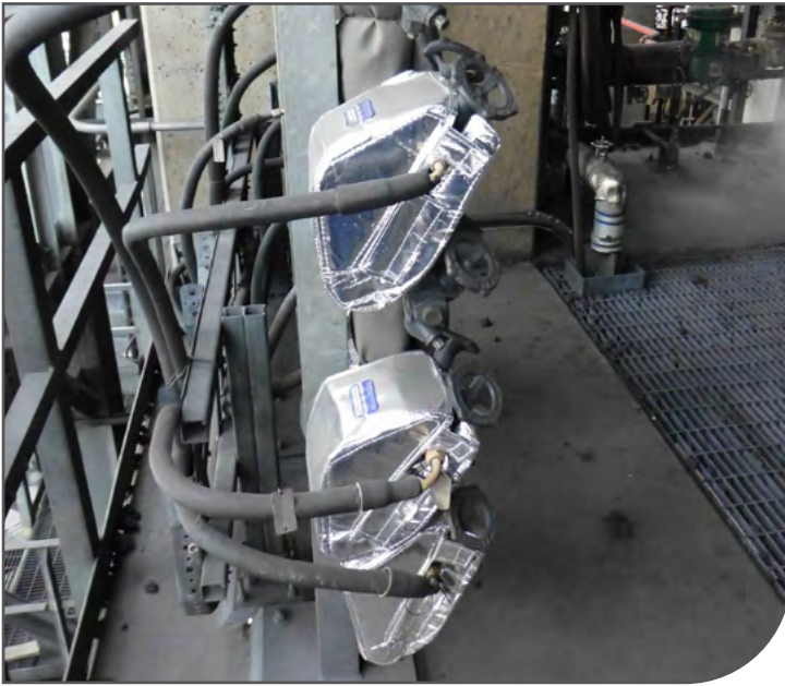
Refinery - Armstrong® Steam Trap / Trap Valve Station Design: LT500HS-AG - 3/32" Thickness Fastener: Velcro Flaps Purpose: Energy Savings & Personnel Protection
