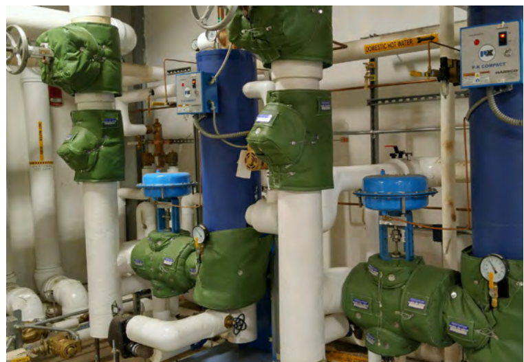
STEAM TO HOT WATER HEAT EXCHANGER Design: LT450TT-1 ½" Thickness Fastener: Stainless Steel Wiretwists / Velcro® Flaps
