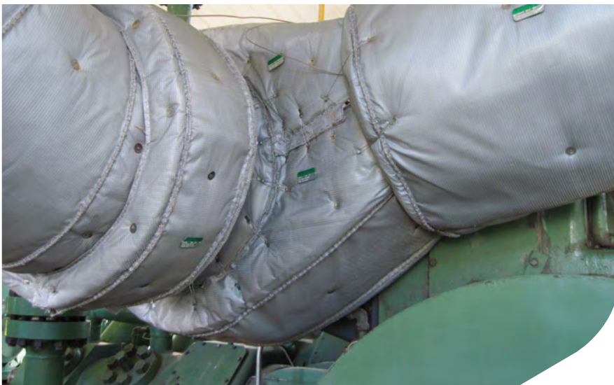
ENGINE DR TLA6 ENGINE EXHAUST TURBOCHARGER Thermal Blanket Design: HT1100MSGM-2" Thickness
