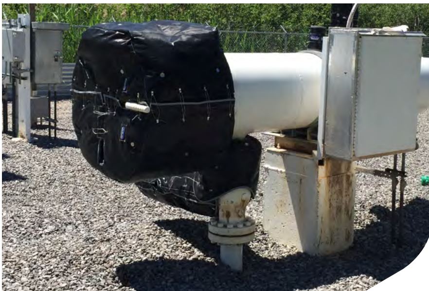
PIG LAUNCHER HEAD
