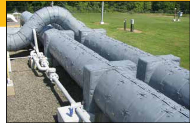
LT450A-TT NATURAL GAS PIPELINE 24" (13 dBA REDUCTION)
