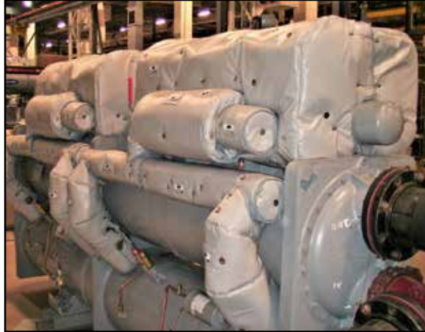
LT250A-VP WATER COOLED LIQUID CHILLER (6 dBA REDUCTION)
