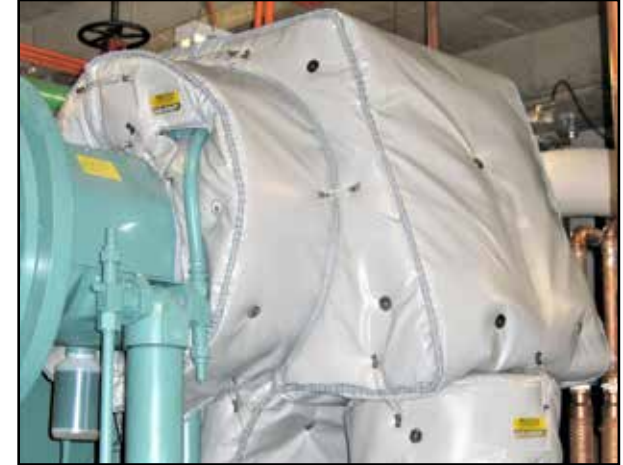
LT250A-VP CENTRIFUGAL LIQUID CHILLER (4 dBA REDUCTION)
