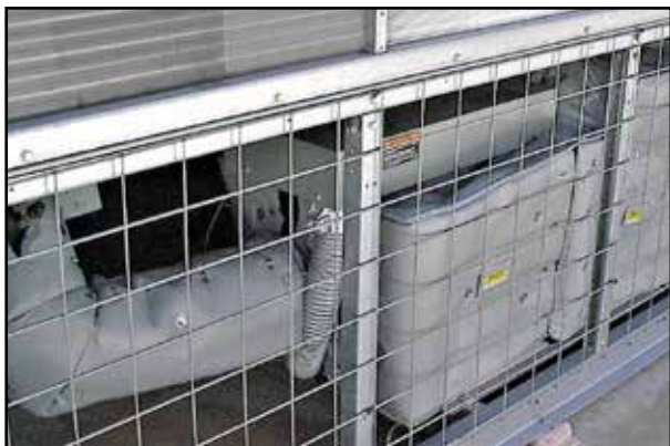
LT450A-TT AIR COOLED CHILLER (6 dBA REDUCTION)
