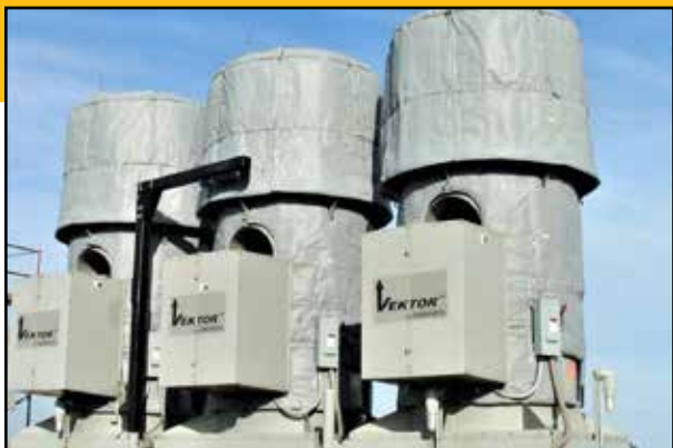
LT450A-TT AXIAL FAN HOUSING (6 dBA REDUCTION)
