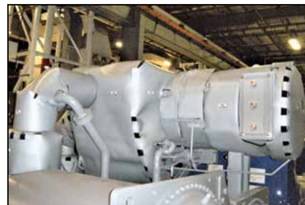
LT250AS CENTRIFUGAL LIQUID CHILLER (6 dBA REDUCTION)
