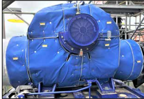
LT400-HES - WIRETWIST, VELCRO FLAP SPLIT CASE PUMP
