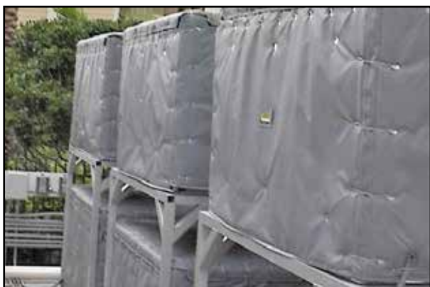
LT450A-TT ACOUSTIC ENCLOSURES (10 dBA REDUCTION)
