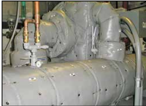
LT250A-VP CENTRIFUGAL LIQUID CHILLER (8 dBA REDUCTION)
